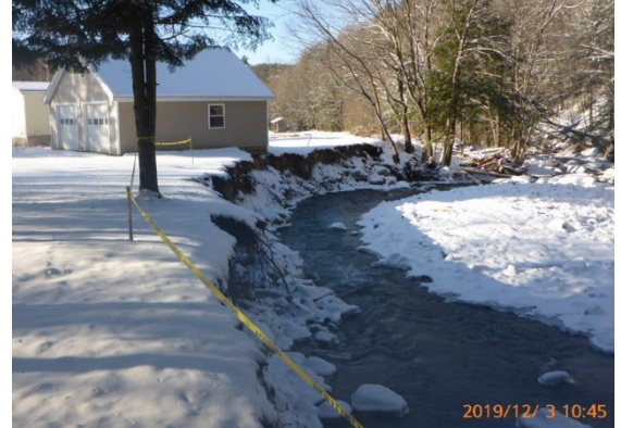
Due to extreme rainfall on October 31, 2019, Lewis Creek in the Town of Bristol, Vermont, had extensive flood flows which caused bank erosion that endangered a two garage and residence.
