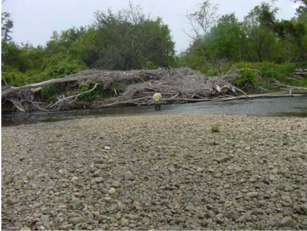
Figure 16: Walloomsac River - Reach M05, Woody Debris and Bar near Route 279 Bridge.
