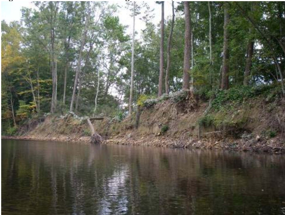
Figure 13: Walloomsac River - Segment M06b, Erosion on Left Bank.
