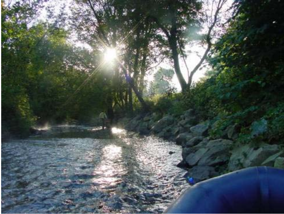
Figure 18: Walloomsac River - Reach M03, Left Bank Revetment, Upstream View.
